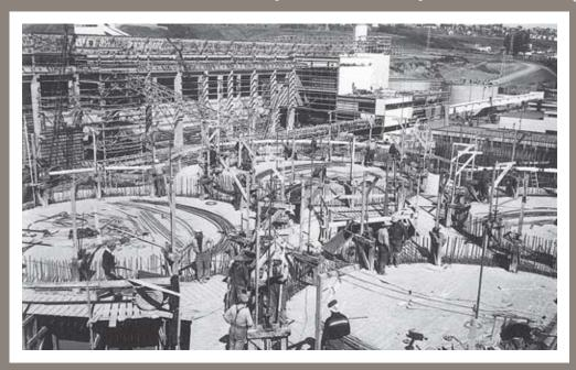
The foundations and boardings for the cement silos in Quebec
