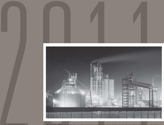
The expanded Wadi plant of ACC in India reached a world record in clinker production with 13,187 tonnes of clinker in one day in February 2011.
