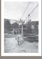
Transport of the raw material with a cable car directly into the production halls.
