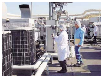
Energy-saving inspection at site
