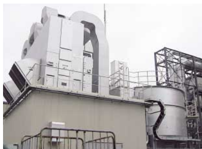
Waste gas combustion facility at Sendai plant
