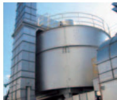
Equipment for the detoxification of VOC effluent gas from gravure printing presses (Sagami Plant)
