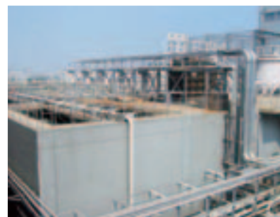
Wastewater recycling system for the treatment of wastewater containing heavy metals and processing to produce purified water (Toppan CFI (Taiwan) Co., Ltd.)
