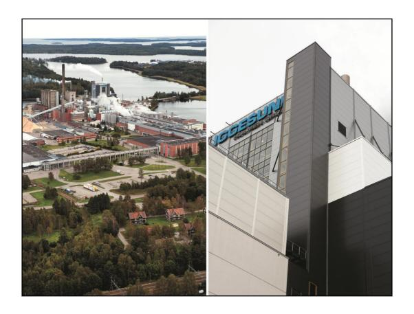
I started off my speech with a few glimpses of the launch and opening of the recovery boiler at Iggesund Mill. Here's a bird's eye view of the mill and, on the right, a close-up of the building that houses the recovery boiler.
