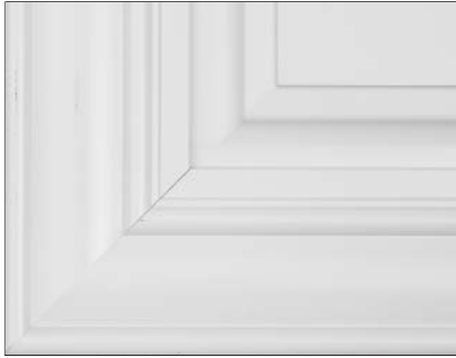
Example of door front joint separation
