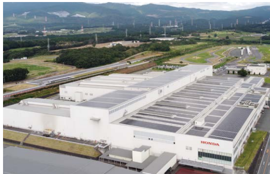
Kumamoto Factory (5.35 MW)
