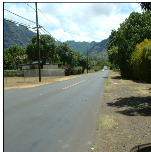
Typical road section along Mākaha Valley Road.
