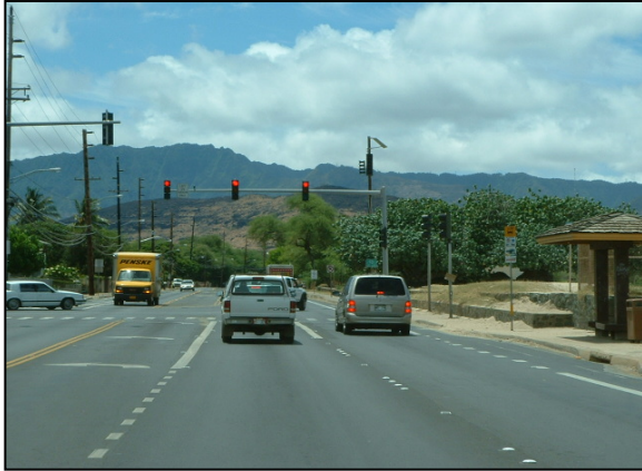
Farrington Highway intersection with turn lanes and overhead electric.
