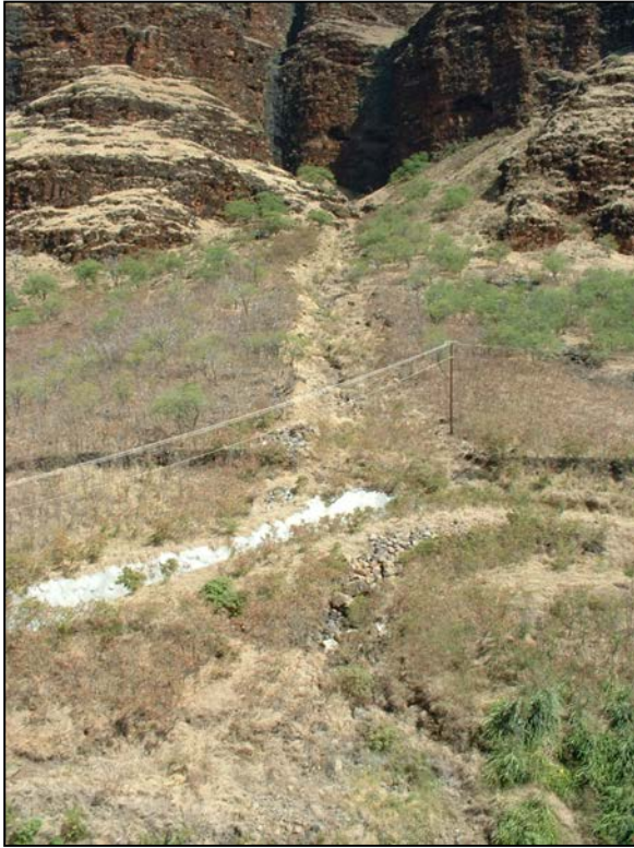
Drainage area behind Mākaha Valley Towers.
