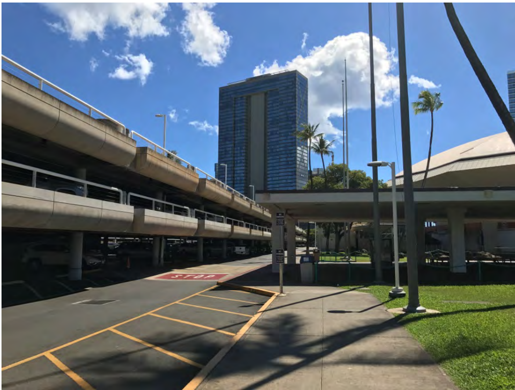
Photo 8. Looking makai from the walkway between the Exhibition Hall and the parking garage (KOP4)
