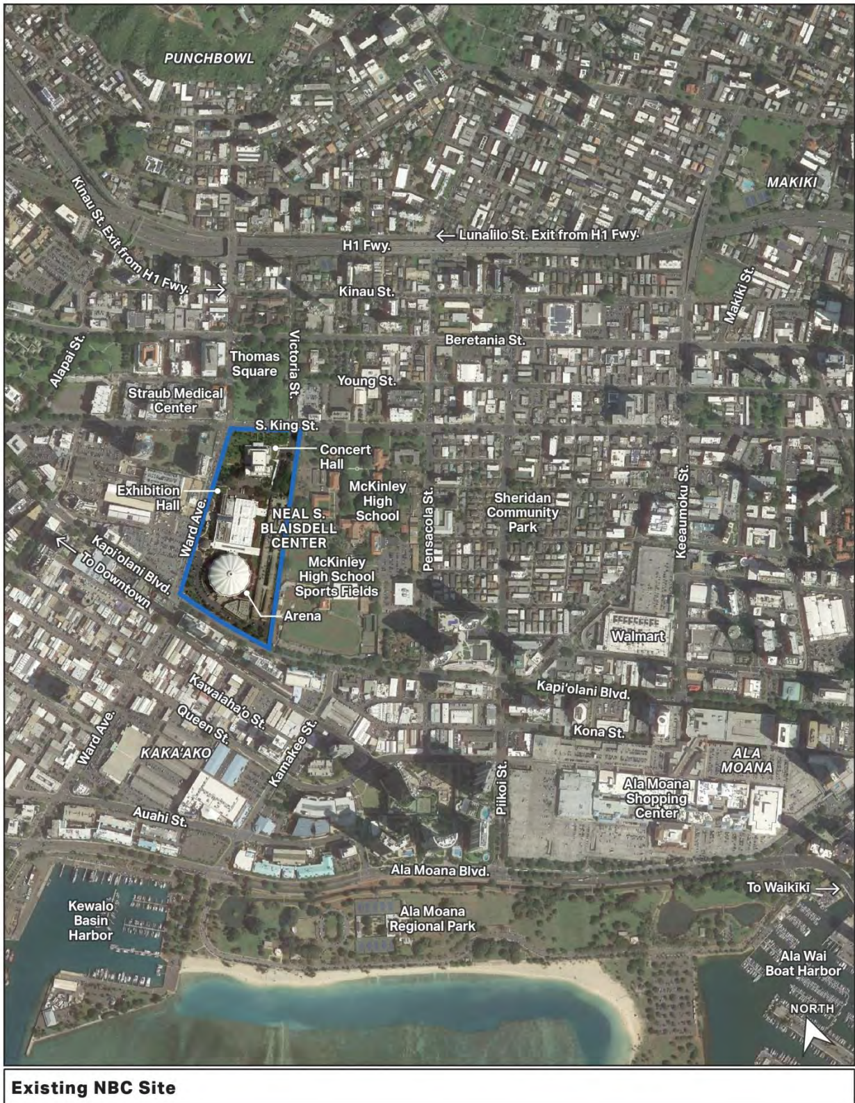
Figure 1: Existing NBC Site
