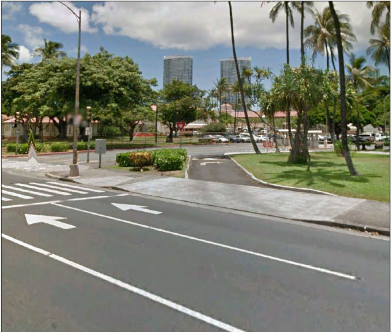
Existing South King Street Channelized Right-Turn Lane into NBC
