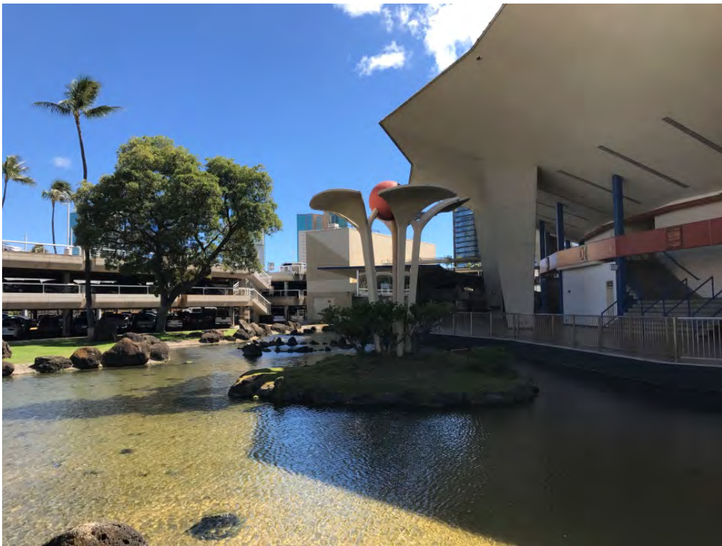
Photo 6. View of the water feature fronting the Arena (KOP3)
