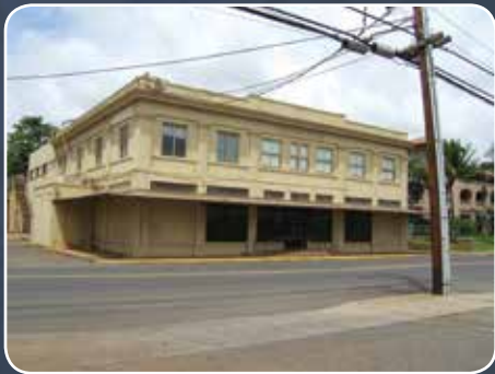
Historic Waipahu Store building
