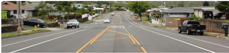
Road diet with two ten foot wide travel lanes, a center-turn lane, two bike lanes and on-street parking in Kailua, Oahu.
