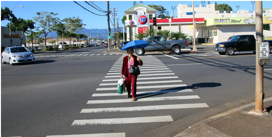
Multi-lane intersections and large corner radii create an uncomfortable pedestrian crossing environment at most California Avenue intersections.
