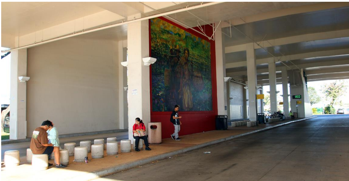
Wahiawa Transit Center and Park & Ride is a major pedestrian trip generator.
