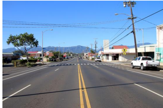
The wide and straight cross section of California Avenue induces drivers to speed and to focus on the road instead of pedestrians.
