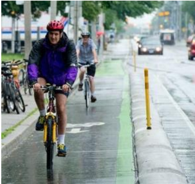
Raised median buffer with green painted pavement in conflict zones in Washington County, OR.
