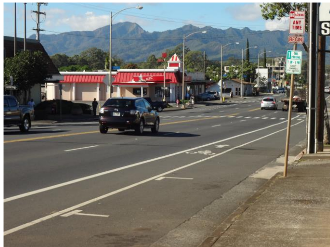
There are many open parking stalls along California Avenue.
