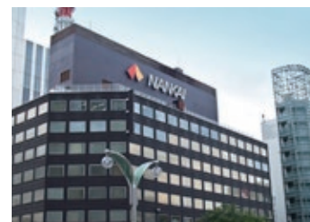
Nankai Tokyo Building
