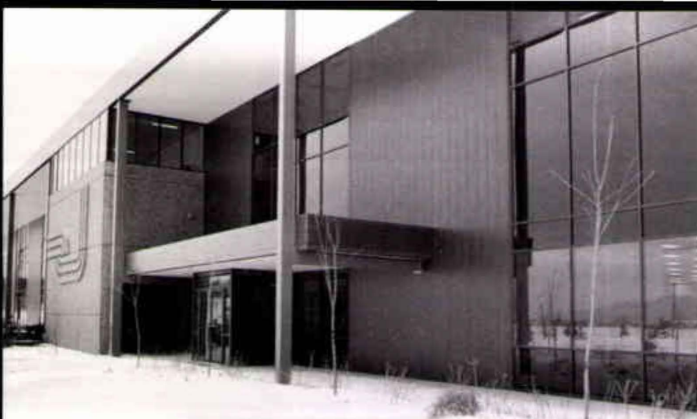
A good portion of Spokane Division will move into this new building in early March, but employment is increasing so rapidly that some departments will remain in the division's two temporary buildings for the next few years.
