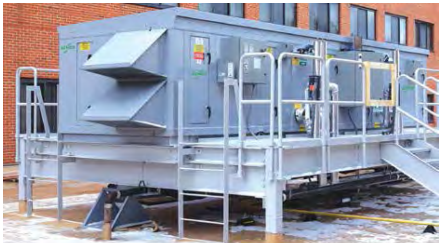
This conventional cooling, active desiccant dehumidification system delivers and controls low dew point air while minimizing regeneration energy input. Designed for hospitals, archival storage and hotels, the AHR Innovation Award winning unit delivers supply air humidity levels as low as 15 grains. Since exhaust heat recovery is not needed, the unit is suited to applications requiring 100 per cent outdoor air.
