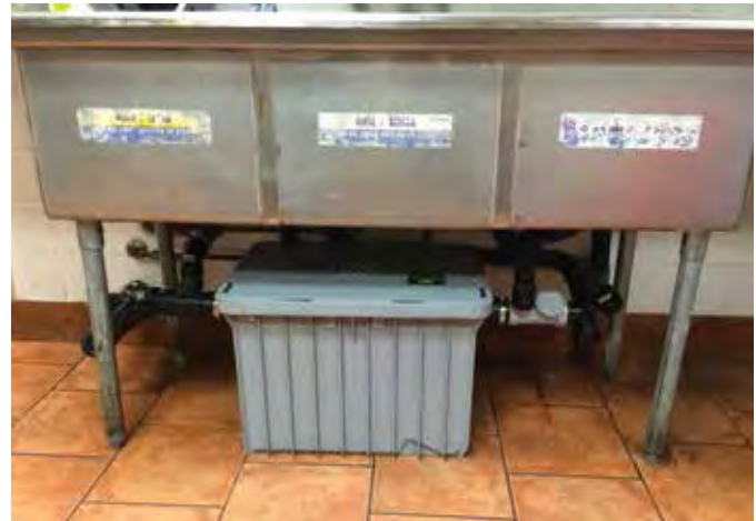
HGIs are generally installed inside the facility they serve, however the market is recognizing the application of Extended Capacity HGI products (up to 100 gpm) that will more commonly be installed outside the building.
