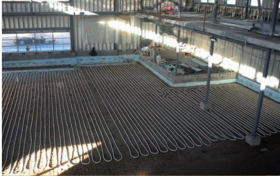
The topmost layer of PEX piping, which makes up the solid thermal energy storage, is shown before the final backfill. The installation was done from "within" the building, before the slab on grade was poured.
