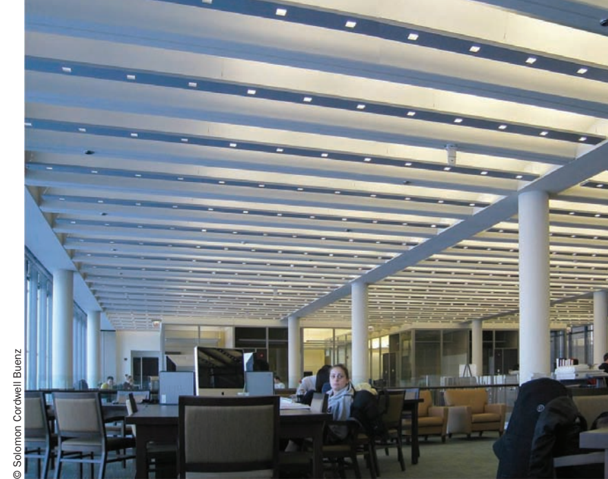
Above Precast concrete panels with cross-linked polyethylene tubing compose the Information Commons’ dual temperature radiant ceilings.
