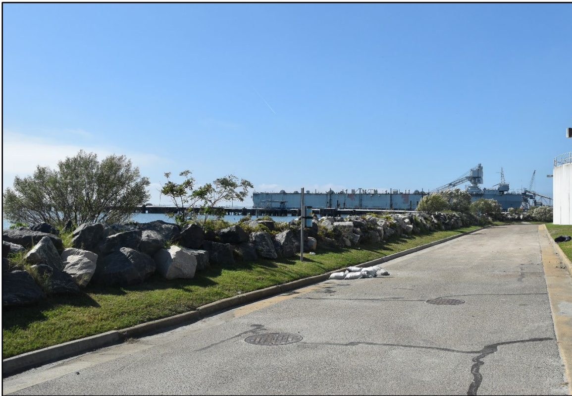
Photograph 1: Pier 15, Looking West (AECOM 2020).
