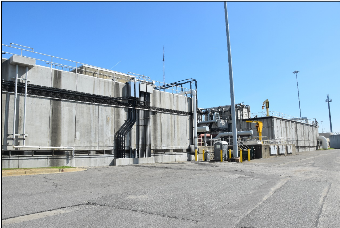
Photograph 4: 1978 Aeration Tanks #1 and #2, Looking Southeast (AECOM 2020).
