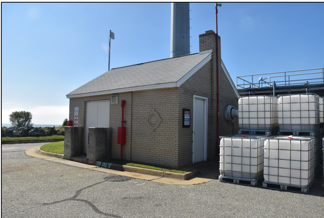
Photograph 5: Jefferson Avenue Pump Station, Looking Southwest (AECOM 2020).
