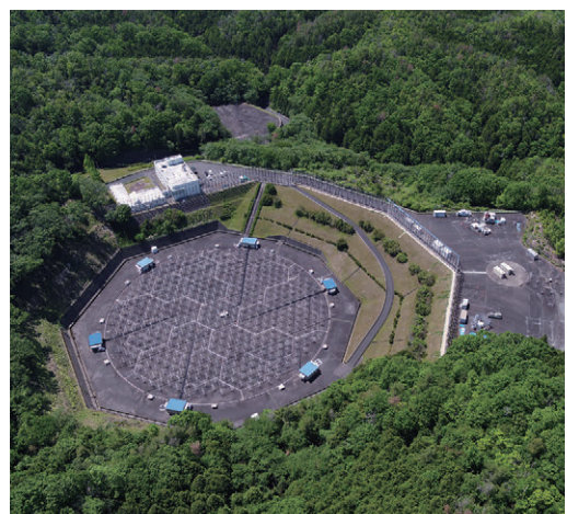
MU radar in Shigaraki, Koka City , Shiga Prefecture. The diameter of the antenna is 103 m.
