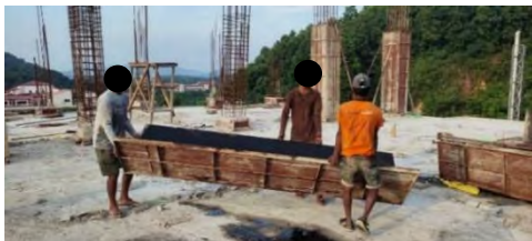
Figure 2. Workers lifting assembled panels to
