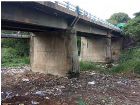
Figure 5. Velanthavalam bridge site
