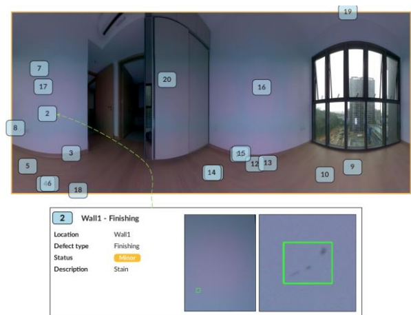
Figure 10. A panoramic visualization showing accurate defect-positions with close-up image.
