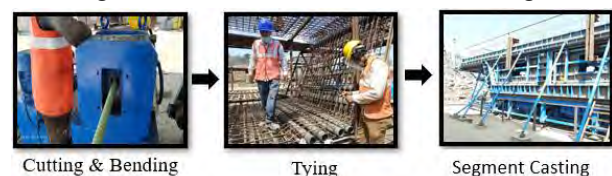
Figure 1. Segmental Production Process
