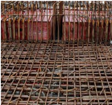
Figure 2. Representative picture of heavy reinforcement taken by the author at a similar construction site.
