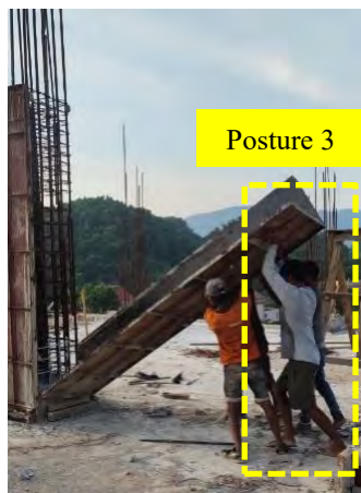
Figure 5. Panel erection
