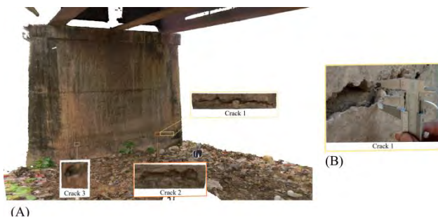
Figure 8. (A) Scanned cracks using TLS (B) Measurement of crack 1 using Vernier scale
