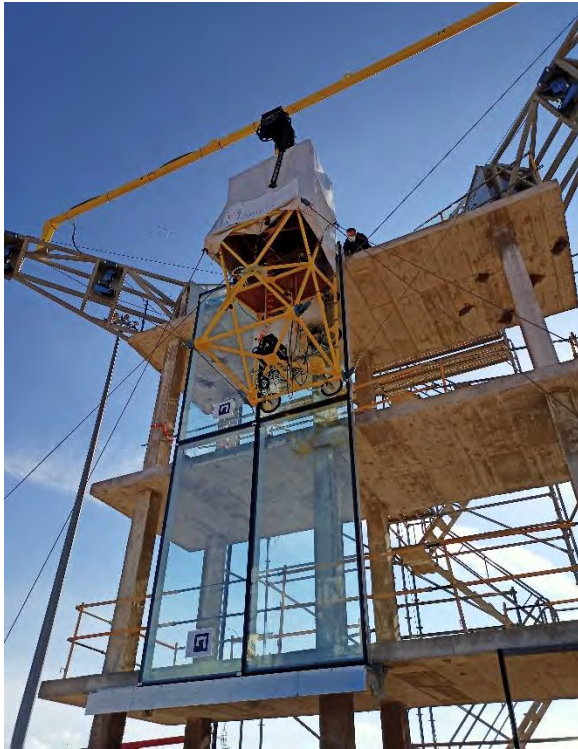
Figure 12. The HEPHAESTUS cable-driven façade installation robot on a testing site (photo: K. Iturralde)
