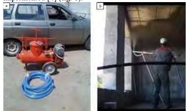
Figure 1. Mobile equipment and technology for applying semi-dry sprayed concrete
