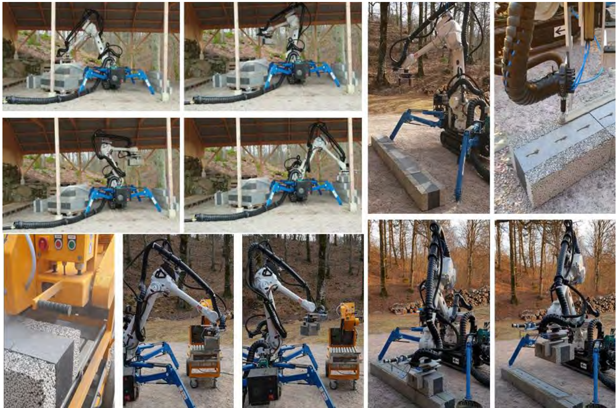
Figure 4. Robotized Finja Exakt processes. a) Wall segment assembly (top left). b) Mortar application (right). c) Sawing (bottom left).
