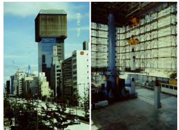
Figure 3. The pioneering automated construction site “SMART” developed by Shimizu Corporation (photo: T. Bock)
