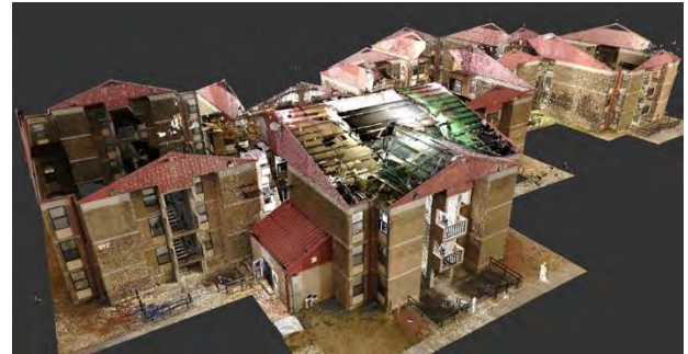
Figure 3. Laser Scanned Model of Building 317 at Ft. Gordon, GA
