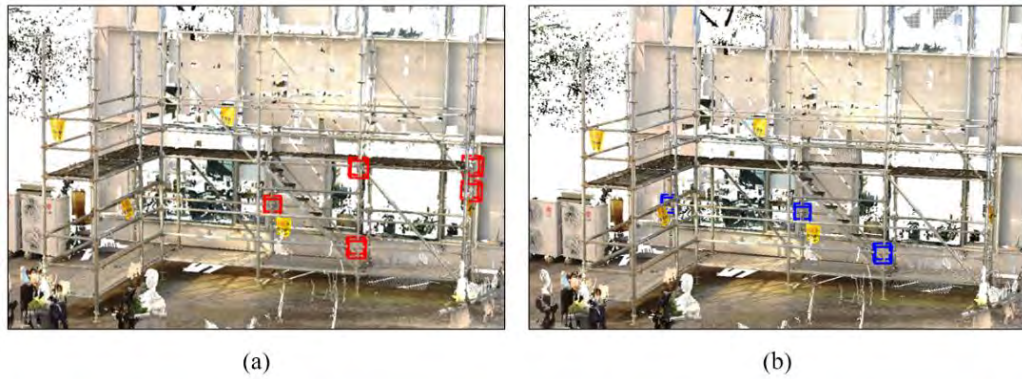
Figure 8. Localization & visualization of unsafe joints; (a) Prediction (red box), (b) Ground truth (blue box).
