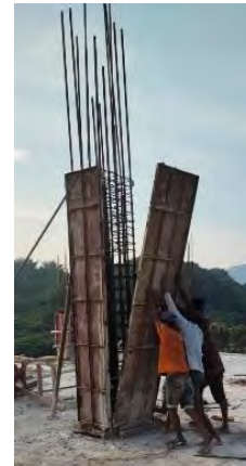
Figure 3. Workers erecting formwork panels around the rebar
