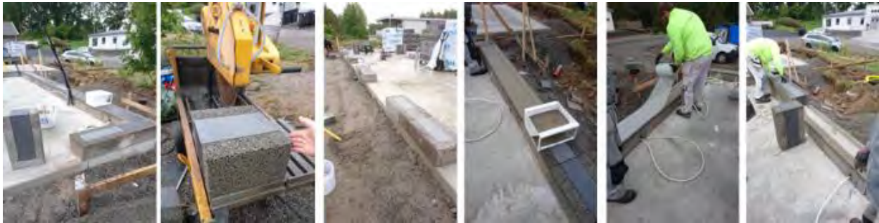
Figure 2. Steps in the manual masonry process in the Finja Exakt block system. From left to right: a) First layer. b) Customization of blocks. c) Door openings. d) Mortar application. e) Reinforcement application. f) Customization for cabling. [12]
