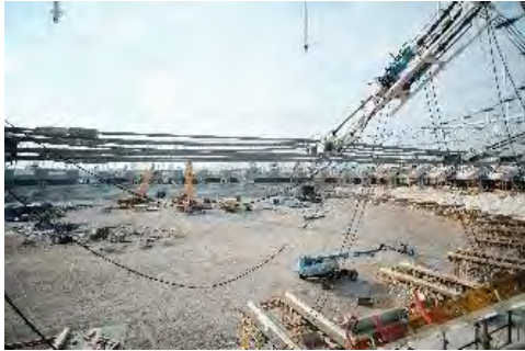
Figure 7 The lifting process
