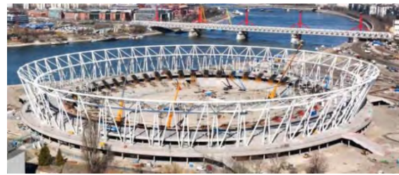
Figure 9 The cable lifting final stage
