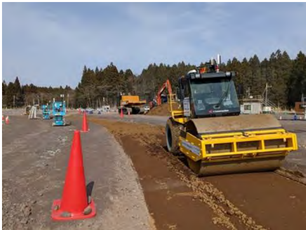
Figure 5. Autonomous heavy machinery fleet for large infrastructure projects (Photo: T. Bock)
