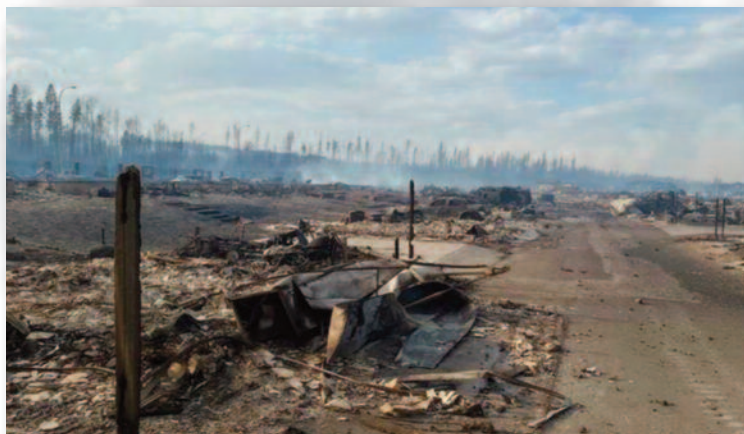
The remains of a Fort McMurray subdivision.
