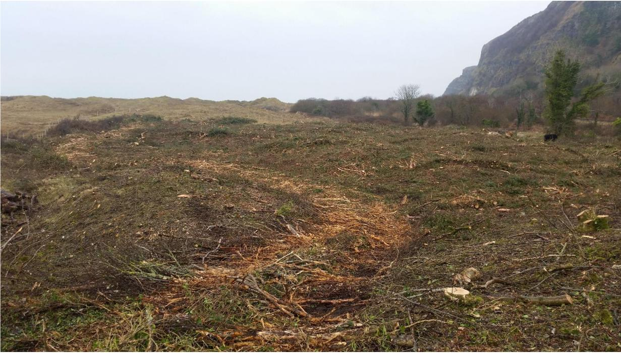
Figure 61: Site cleared ca 15 days. Note brash and waste wood remain on site. Next phase of site clearance commences.
