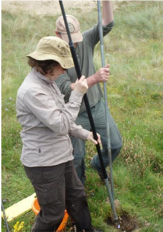
Figure 70: Piezometer Installation.
