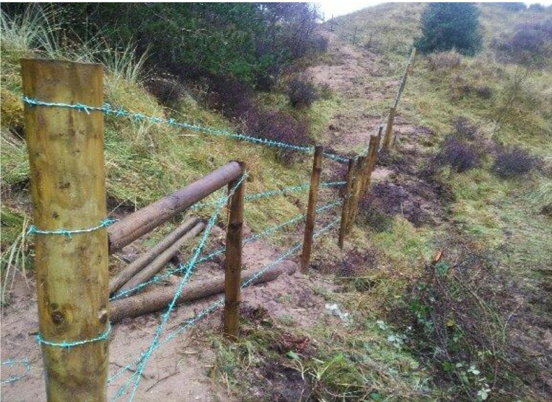
Figure 50: Stock proof fencing installation to facilitate conservation grazing.
