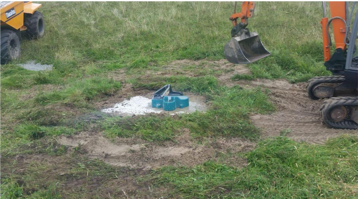
Figure 66: Pasture pump – one of 4 across the site, utilising groundwater for cattle. Access Umbra burn closed.
