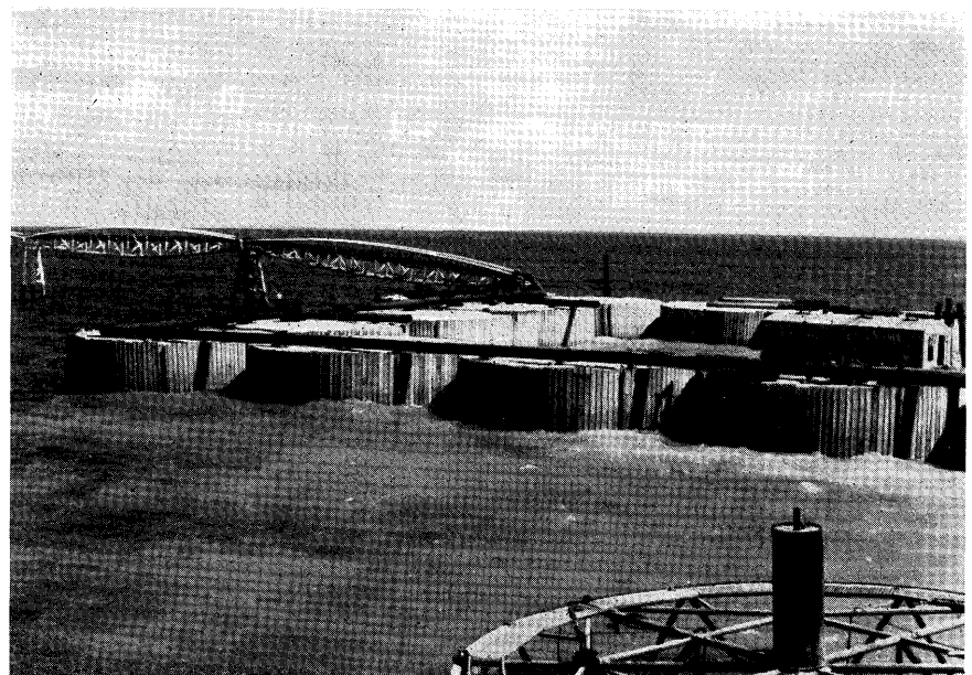
2. Circular sheetpile cells form the perimeter of the island.
