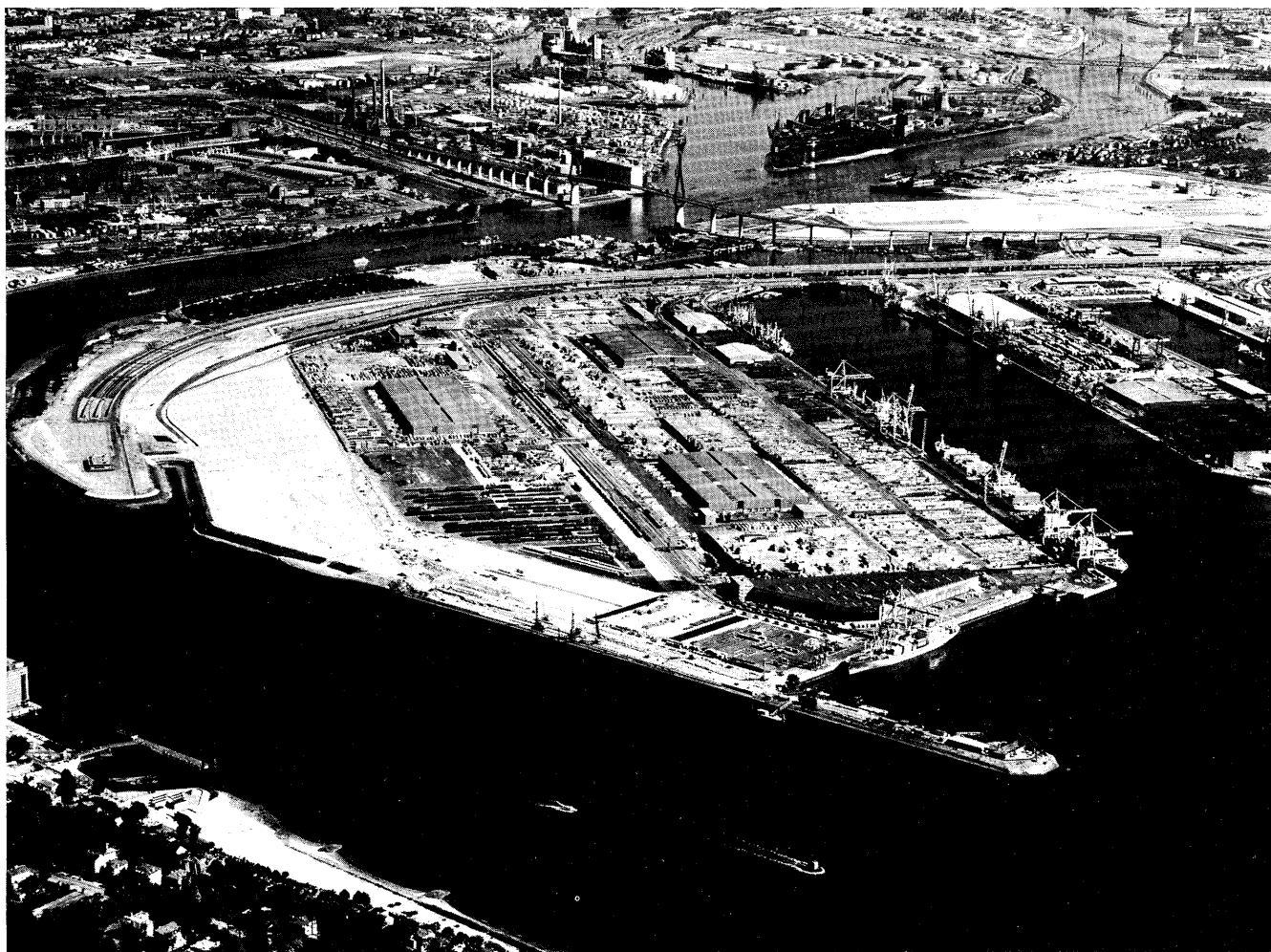
Hamburg Container Center is being readied for South-African container service.
