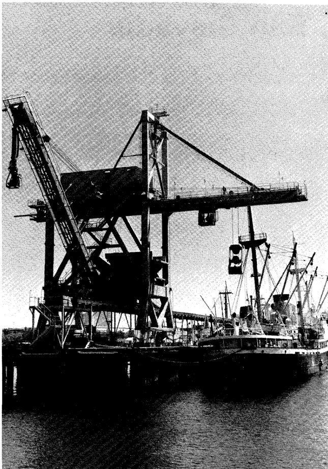
Loading unit—Port of Acajutla
