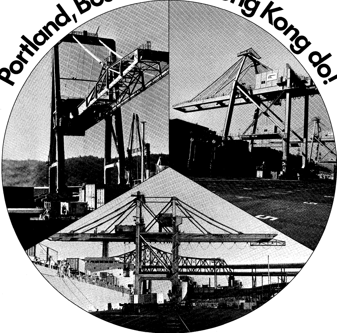
Container cranes supplied to the Port of Portland, U.S.A.
