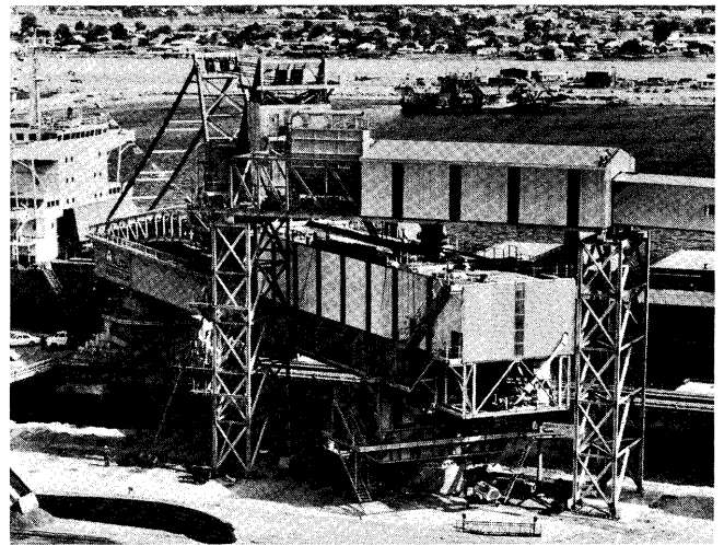
Fig. 11—The transfer station between the dock conveyor and Linear Loader is a fixed structure, that can be completely enclosed and sealed, incorporating extensive dust control installations.
