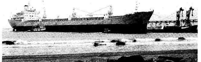
Maritime terminal of Salaverry. A partial view of the wharf.
