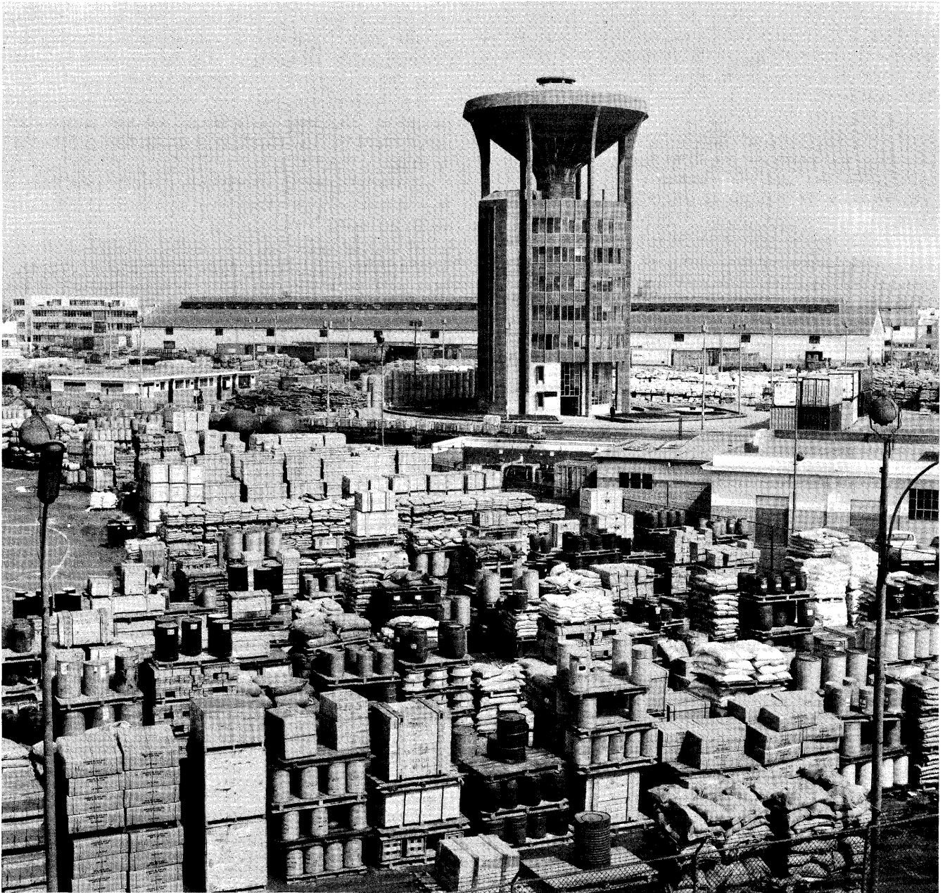
Maritime terminal of Callao. Storage Zone 1 and the administrative building.
