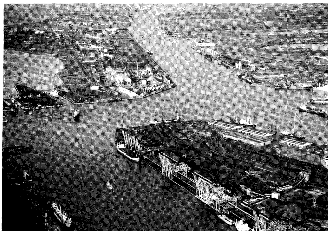
Antwerp:—"Stocatra" ore transshipment plant, new canal dock and twin locks.
