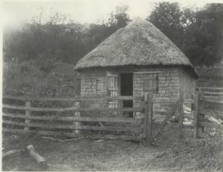
2. Protective structures over mosaics at Great Witcombe, Gloucestershire, erected 1819 and subsequently modified (© Crown copyright, NMR).
