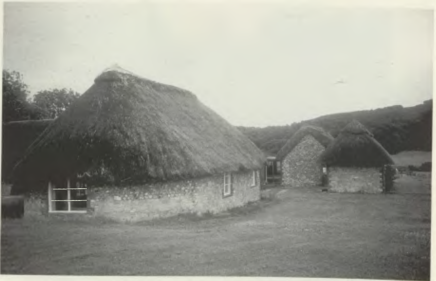
6. Bignor Roman Villa, the protective structure over the Venus mosaic, erected soon after its discovery.
