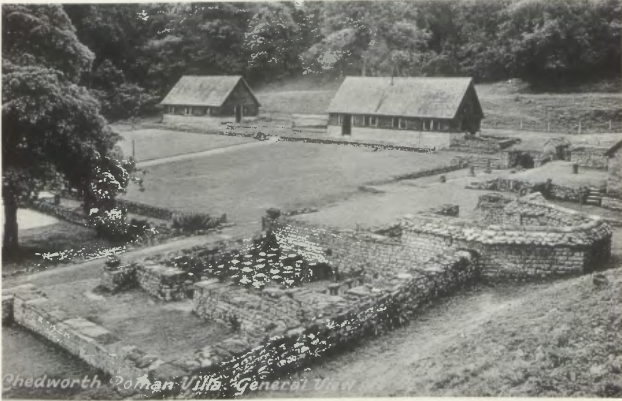
3. Chedworth Roman Villa, Gloucestershire, first half of the twentieth-century, general view of protective structures over mosaics.
