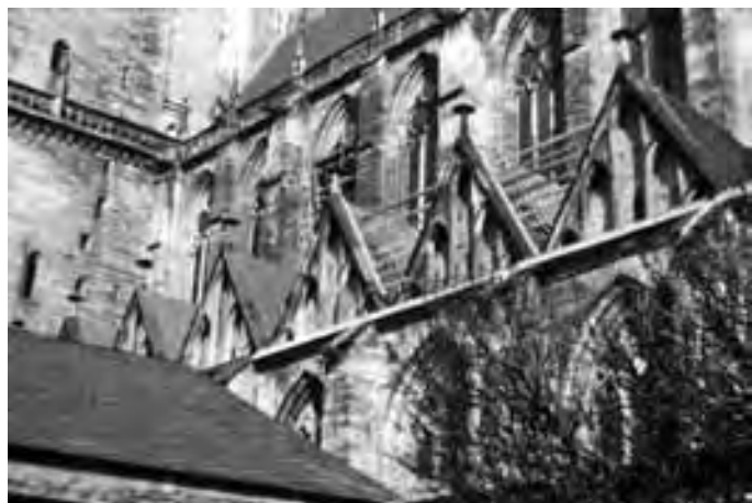
Figure 183. Magdeburg Cathedral, south aisle gables in 1979
