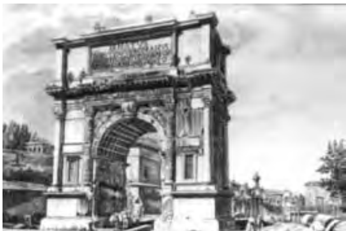
Figure 109. Arch of Titus: the side toward the Colosseum after restoration (Rossini)
