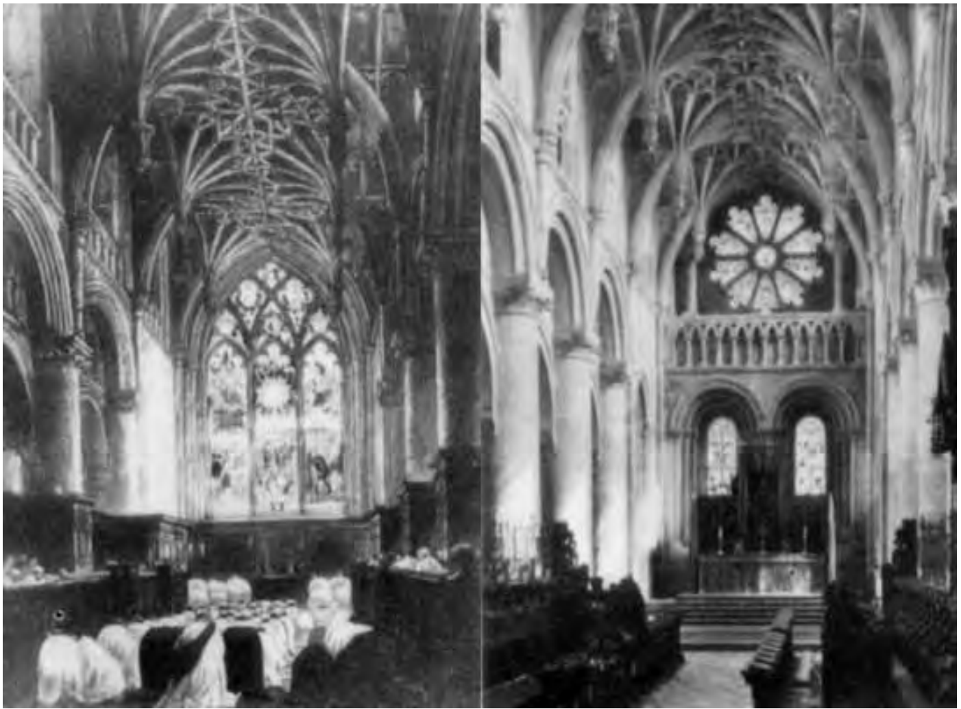
Figures 291 and 292. Oxford Cathedral: the east end before and after restoration by Scott
