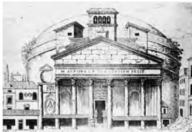
Figure 54. The Pantheon in the early 17th century. Two columns and three capitals of the portico are missing. The pediment is broken; a bell tower marks its use as a church
