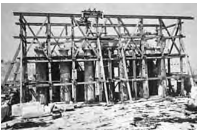
Figure 134. The Propylaea under restoration, c. 1900
