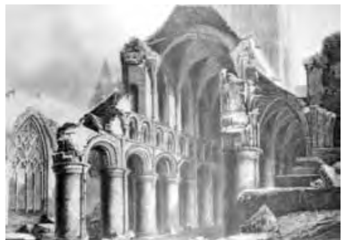
Figure 267. Hereford Cathedral after collapse in 1786
