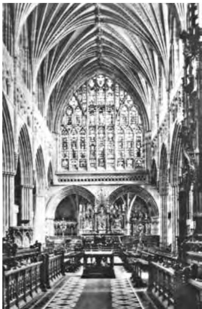
Figure 277. Exeter Cathedral with the reredos restored by Sir George Gilbert Scott
