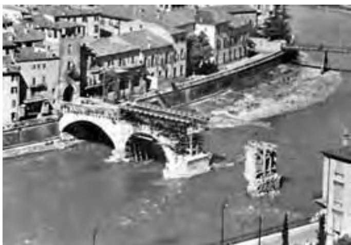
Figure 337. Ponte Pietra in Verona, being reconstructed after the Second World War destruction
