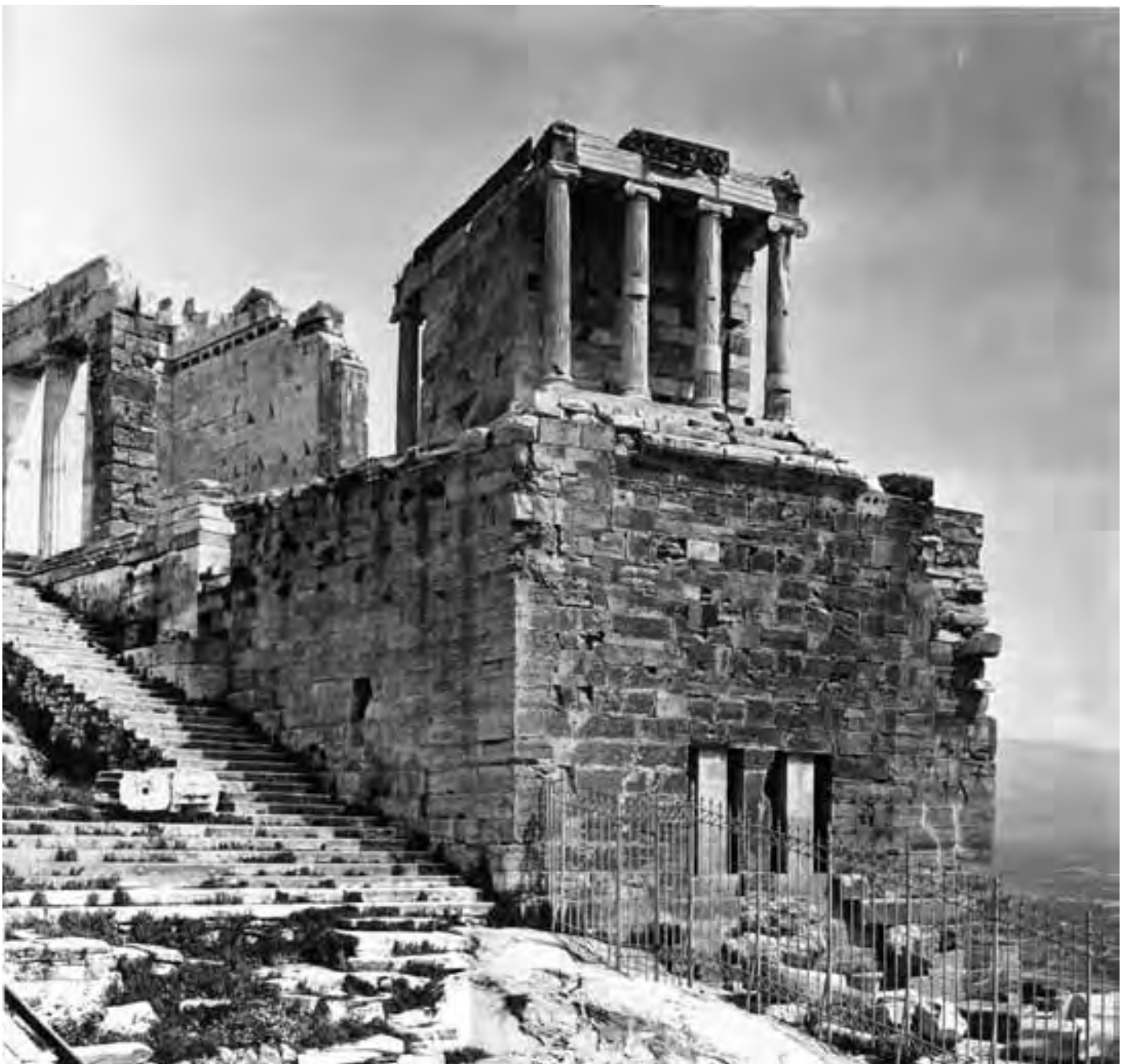
Figure 125. The Temple of Athena Nike c. 1900. The basreliefs have been replaced with terracotta copies from the originals in the British Museum (Elgin Marbles); losses have been integrated in simple forms with no details
