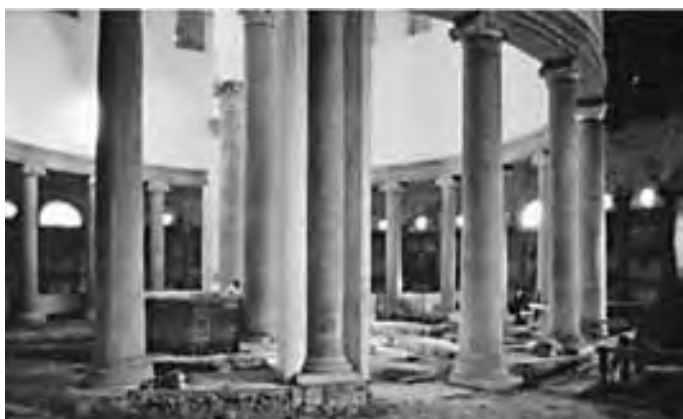
Figure 19. The interior of the church of S. Stefano Rotondo, Rome
