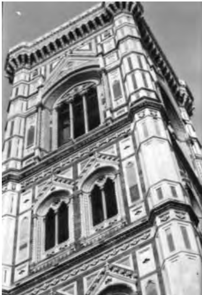
Figure 287. Detail of Giotto's Bell Tower in Florence
