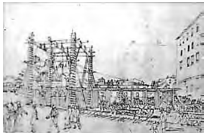
Figure 94. The Temple of Vespasian and Titus, Forum Romanum, Rome. Dismantling of the architrave 1810-11
