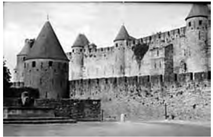
Figure 260. Carcassonne, Le Cité after restoration, photo in 1980
