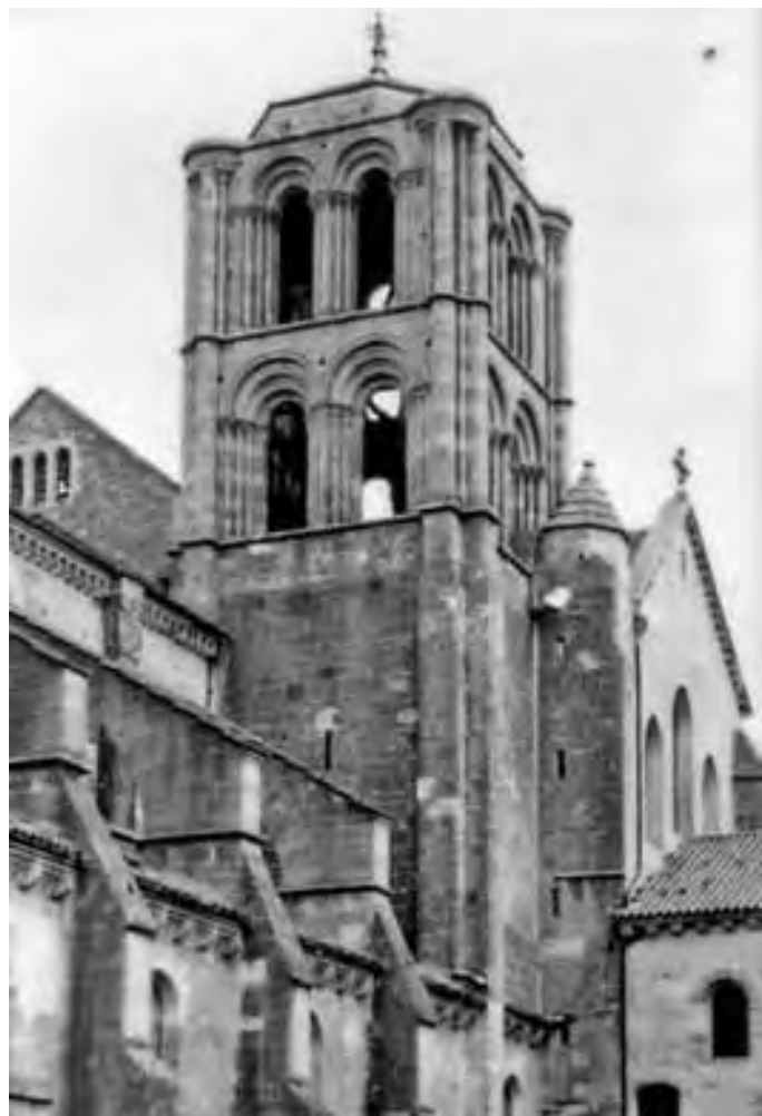
Figure 197. La Madeleine, the transept tower in 1980
