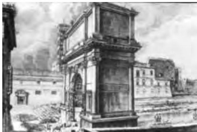
Figure 110. Arch of Titus: the side toward the Forum after restoration (Rossini)
