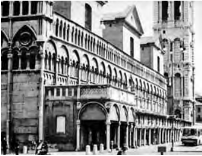
Figure 344. Ferrara Cathedral with the small shops on the south side possible removal of which was discussed with the purpose to display the entire church elevation
