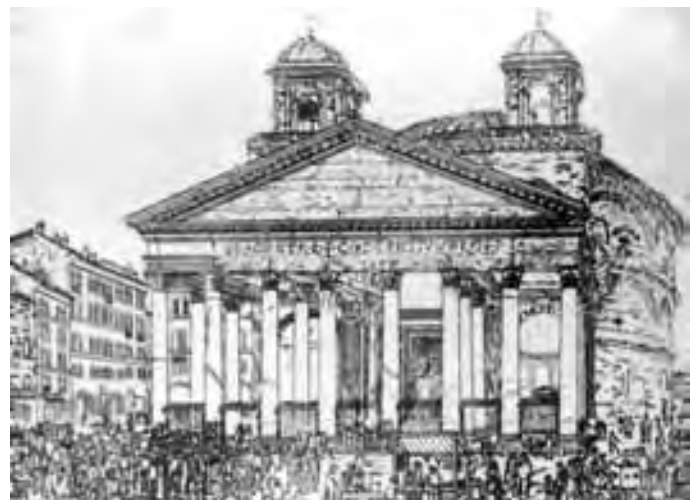
Figure 55. The Pantheon after the 17th-century restorations. Urban VIII ordered the dismantling of the bronze vault of the portico, and the construction of two new bell towers. Alexander VII ordered the restoration of the portico
