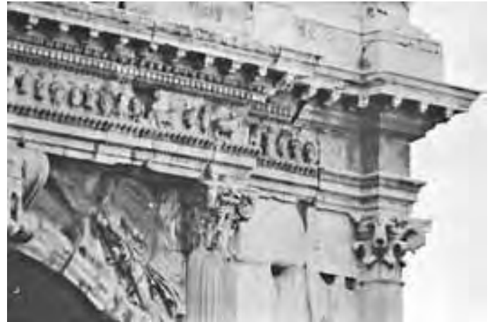
Figure 108. Arch of Titus, detail showing the distinction between original (in marble) and new (in travertine and simplified details)
