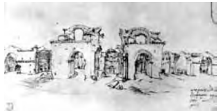
Figure 38. The entrance to the Thermae of Diocletian, Rome, where Michaelangelo built the church of S. Maria degli Angeli
