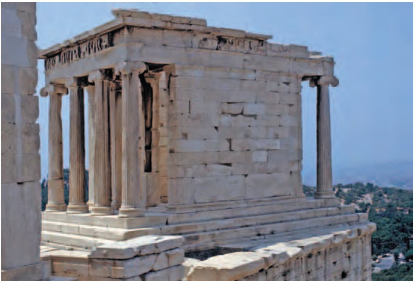
Figure 135. The Temple of Athena Nike after the second reconstruction in the 1930s. Missing elements have here been produced as replicas from the originals. The bas-reliefs in British Museum have been replaced with casts in white cement (photo in 1980s)
