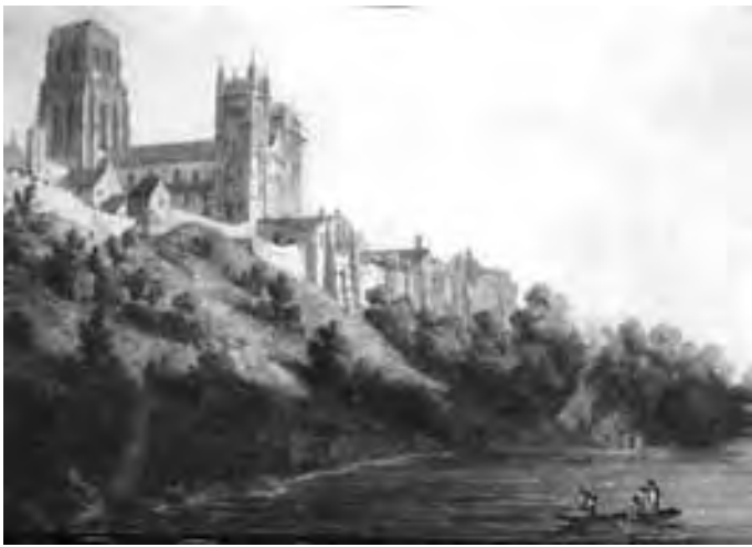
Figure 140. Durham Cathedral. Detail of watercolour by E. Dayes in 1795, showing the scaffolding for the construction of the pinnacles
