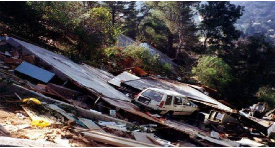
Figure 4. Hillside building collapse in the 1994 Northridge, California Earthquake (Credit: City of Los Angeles Department of Building and Safety).
