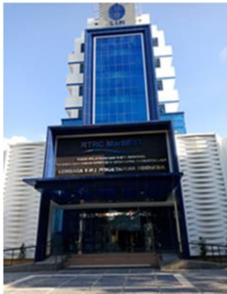
Figure 21. RTRC-MarBEST Building at Jalan Raden Saleh
