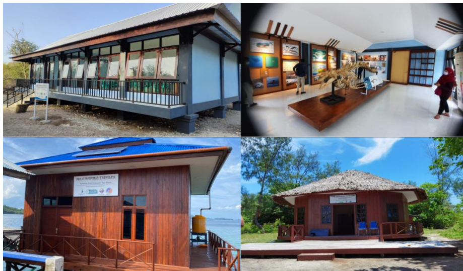
Figure 33. Infrastructures built by subgrantee. Upper left and right: Information center in Oesina, Kupang; Lower left: Information center in Yellu, Misool; Lower right: Information center in Small Meosarar
