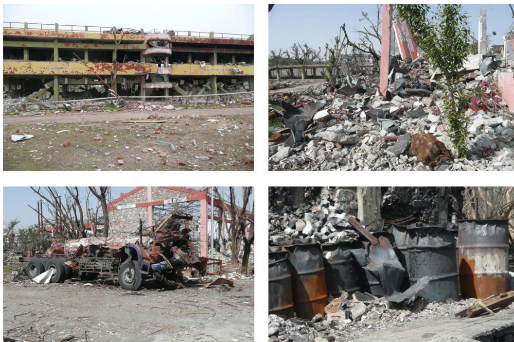
Figure 2. Examples of Onsite Pressure Damage
