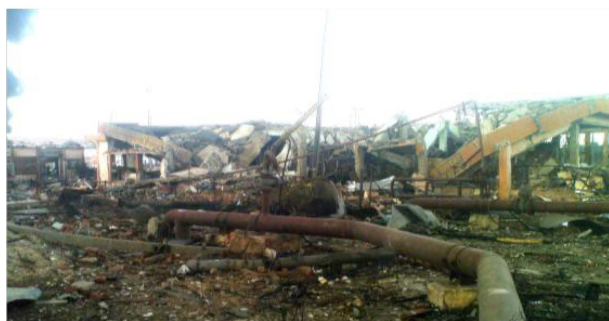
Figure 6. Control Room in Pipeline Division Area (top picture from north, bottom picture taken from south)
