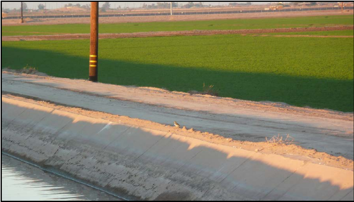
PHOTOGRAPH 7 View of North-south Concrete-lined Canal, Facing Northeast
