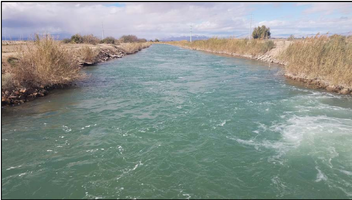
PHOTOGRAPH 6 View of Westside Canal, Facing West.
