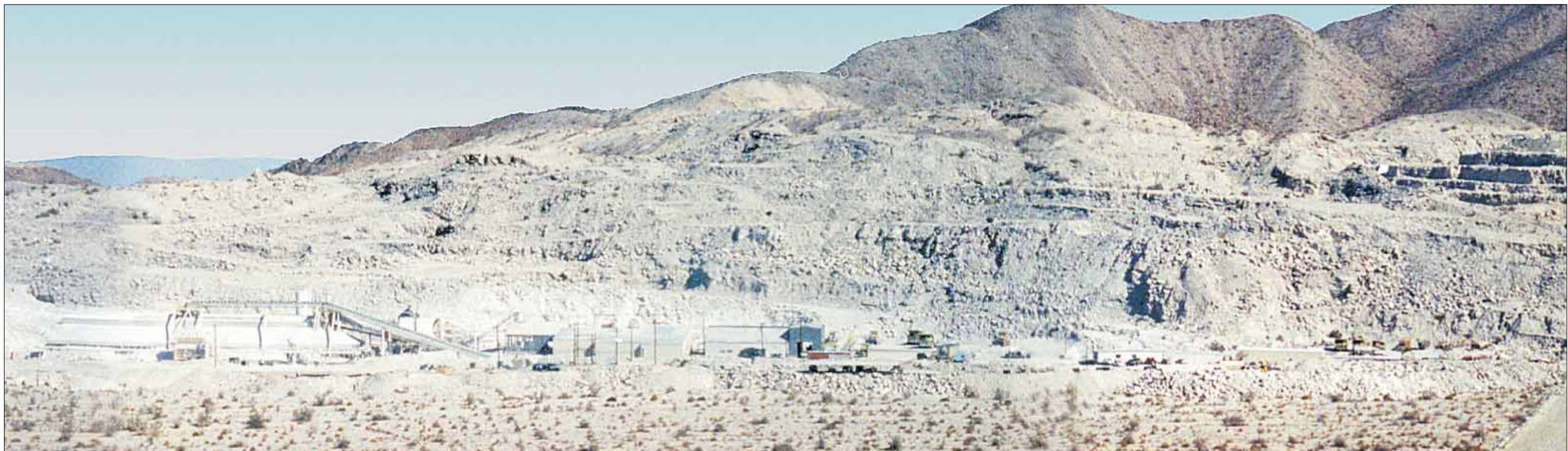
Photograph 5: Plaster City Quarry Plant looking east with Quarry 1B in background.
