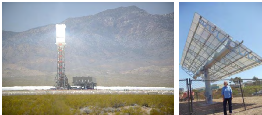
Figure 5. A) Ivanpah's Solar Electric Generating Facility (CSP); B) A CPV Tracker by Soitec
