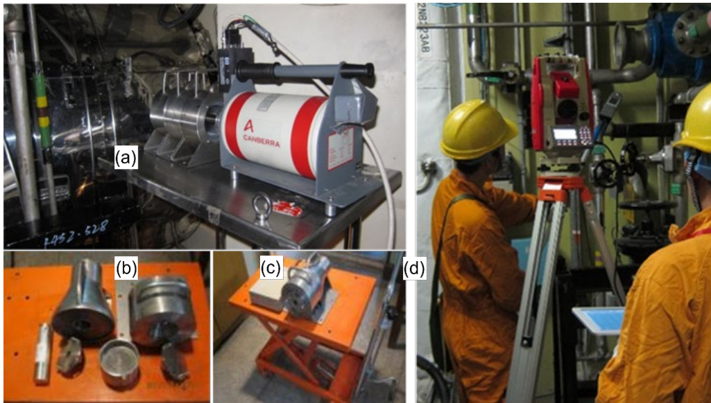
Fig. 3. Radiological on-site measurement. (a)(b)(c) HPGe detector-based gamma radiation source term measurement system and (d) total station for coordinate measurement.
