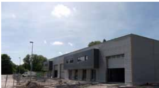
Hall-relais de Manage-Scailmont
