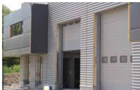
Hall-relais de Manage-Scailmont
