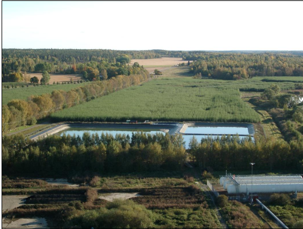
Figure 4: View of the Enköping municipal wastewater plant in Sweden, showing the water storage ponds and willows used as vegetation filter. A 75-ha willow plantation treats and utilizes decanted water from the dewatering of sewage sludge. The water contains approximately 25% of the N entering the wastewater treatment plant, but less than 1% of the water volume. By treating the water separately in the willow vegetation filter, instead of pumping it back into the treatment plant, the total N load is reduced by 25%. The biomass produced is used in the local district heating plant, contributing to the local supply of heat and electricity. Ash from the boiler is recycled back to the willow plantation. Photo credit: Per Aronsson, Swedish University of Agricultural Sciences, Sweden.
