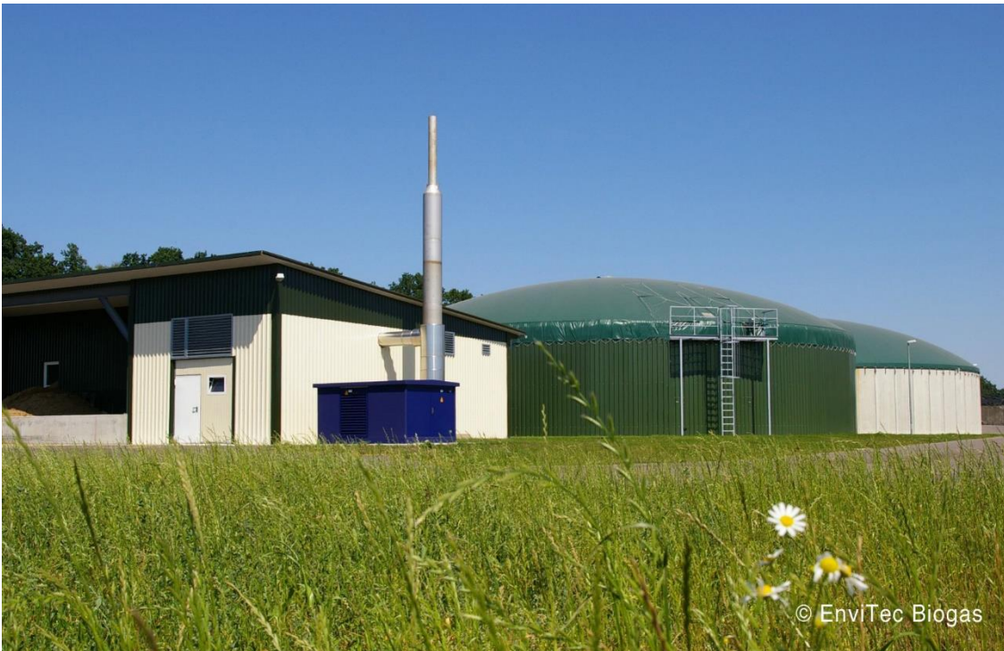
Figure 1: EnviTec biogas plant (Source: EnviTec Biogas AG)
