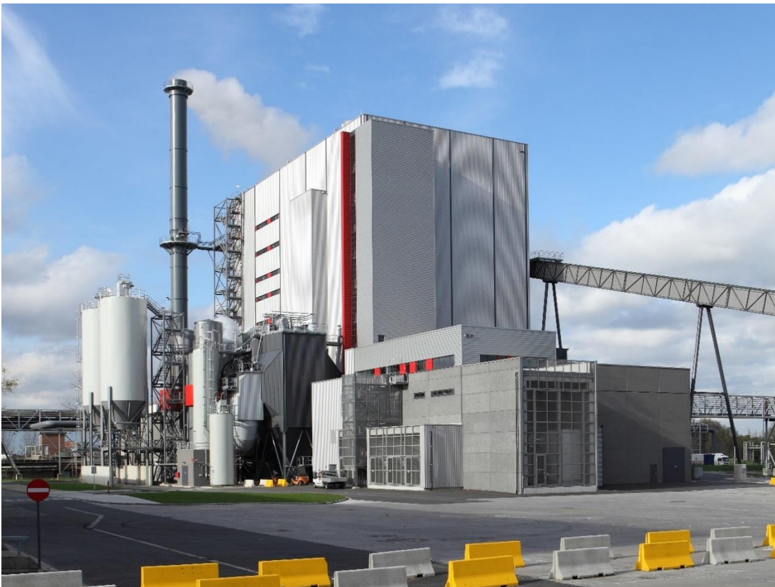
Figure 3: Stora Enso Langerbrugge utilizes renewable energy in paper production. Technology: Valmet CFB Boiler (circulating fluidized bed boiler) (Source: Valmet Oyj)
