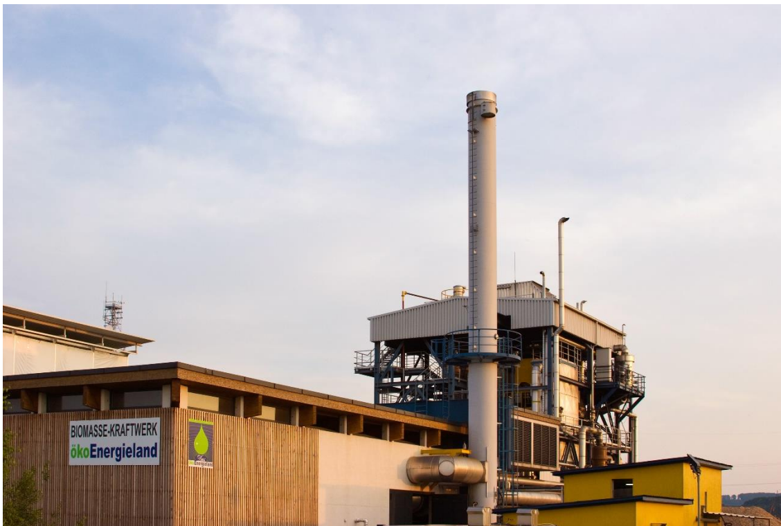
Figure 4: Güssing Dual Fluidized Bed Steam Gasifier, Austria (Source: Bioenergy and Sustainable Energies GmbH)
