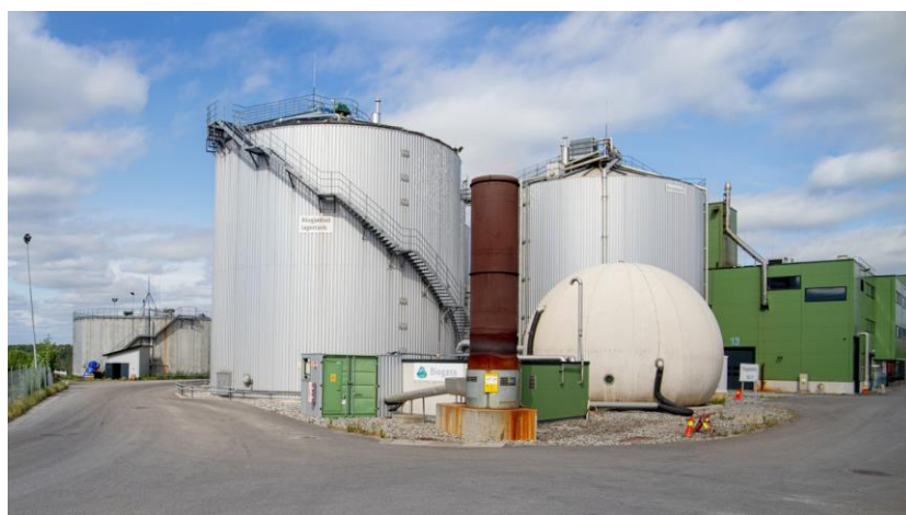
Figure 13.6. Oslo biogas plant Romerrike processing food waste to bus fuel and fertilizer
