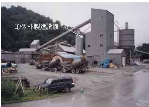
Photo 3 A Concrete Production Facility Housed in a Building
