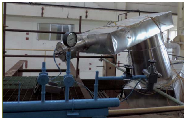
Fig. 1 Gate valve and shield plug on test vessel-2
