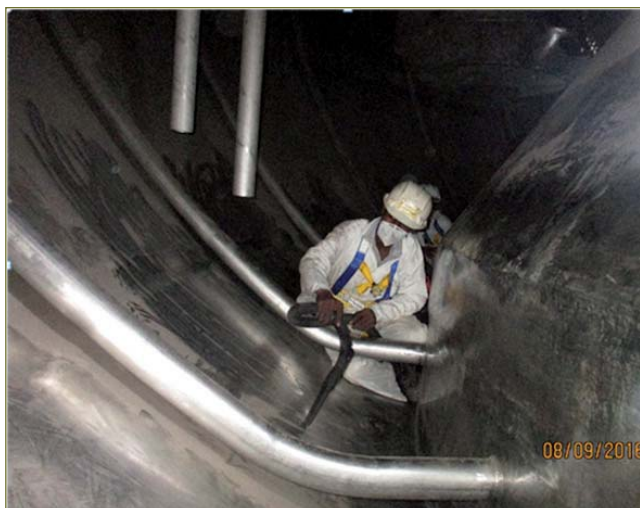
Fig. 2 Vacuum cleaning of cold pool zone of the main vessel
