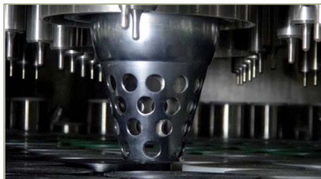
Fig. 4 Core flow monitoring mechanism and thermowells above core top
