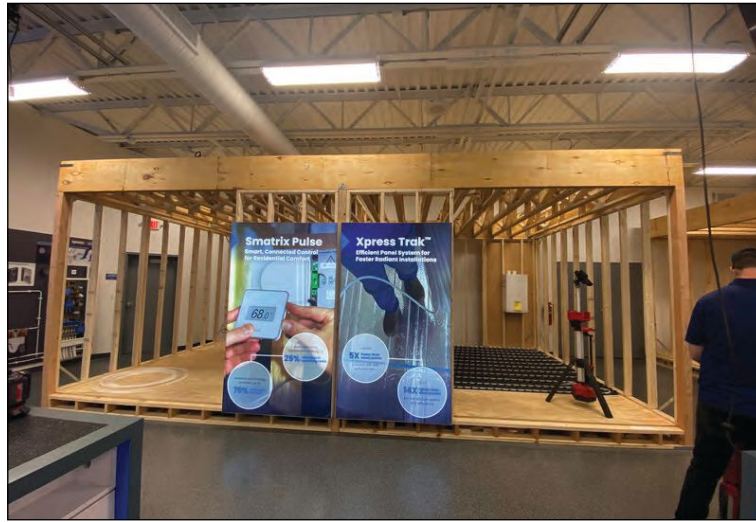
A LOOK INSIDE OF UPONOR'S NEW EXPERIENCE CENTER IN MINNESOTA.
