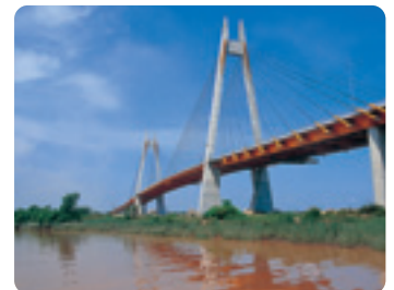
Binh Bridge after completion
