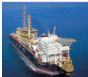
Floating LPG production, storage, and offloading facility
