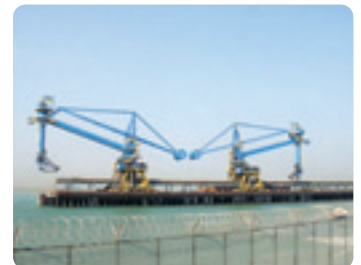
Iron Ore/Coal Continuous Ship Unloaders
