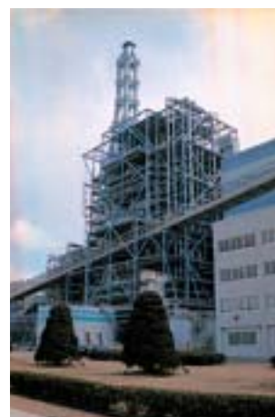
Experimental facility for 360-MW coal-fired combined-cycle power plant for PFBC boiler
