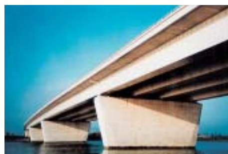
Inabe River Bridge, one of the longest precast, prestressed concrete deck bridges in Japan at 373.5 meters
