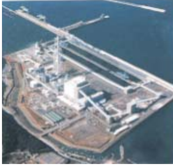
Boilers for power plants
