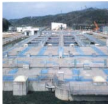
Sewage treatment systems
