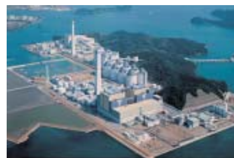
No. 1 Unit of Tachibana-wan coal-fired thermal power station
