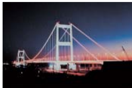
Suspension bridge with 750-meter main span crossing the Irtysh River in Kazakhstan
