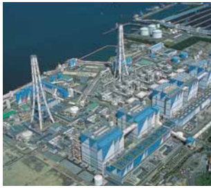
Boilers for power plants
