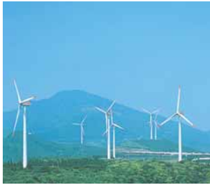
Wind power generation systems
