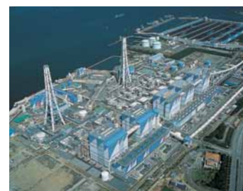
Hekinan Thermal Power Plant of Chubu Electric
