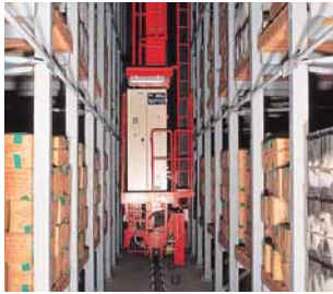
Automated warehousing systems
