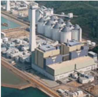
Boilers for power plants
