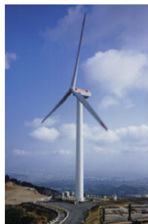
Large-scale wind-turbine generator
