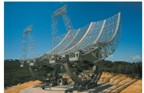
Three-dimensional digital photogrammetry was used on site to verify the correct installation of Tohoku University's synchrotron radio telescope.
