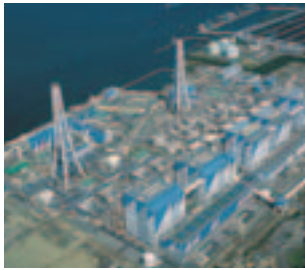
Boilers for power plants
