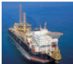
Floating LPG production, storage, and offloading facility
