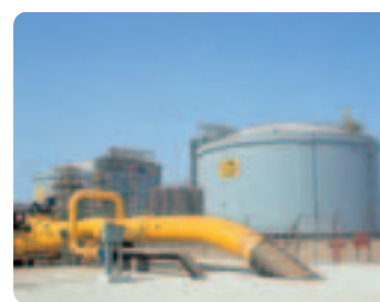
LNG receiving terminal built in India
