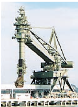
2,700-ton-per-hour continuous ship unloader for coal at Tachibana-wan coal-fired power station
