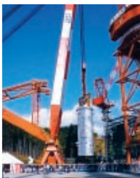
Installation of RPV for Unit No. 3 of Onagawa Nuclear Power Station
