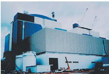
Unit No. 1 of Tachibana-wan coal-fired thermal power station
