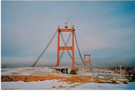
Nearly completed suspension bridge crossing the Irtysh River in Kazakhstan
