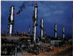
LPG plant for Algeria
