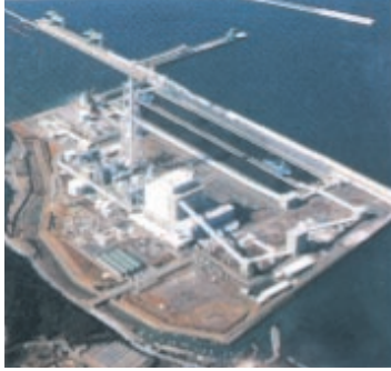
Boilers for power plants
