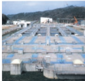
Sewage treatment systems
