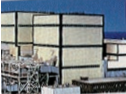
Variable-pressure operated boiler
