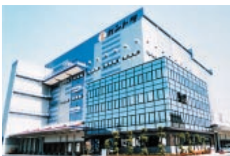
Refrigerated storage automated warehouse system for a subsidiary of Meiji Milk Products Co., Ltd.
