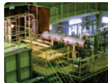
Subzero heat storage system
