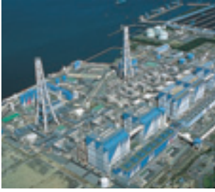
Boilers for power plants
