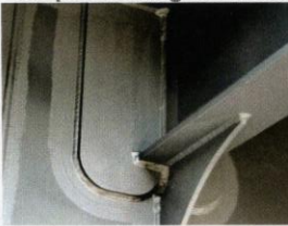
Stripe Coating on Weld
