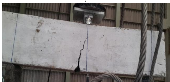
Figure 17: Failure pattern of Steel 1x6 beam
